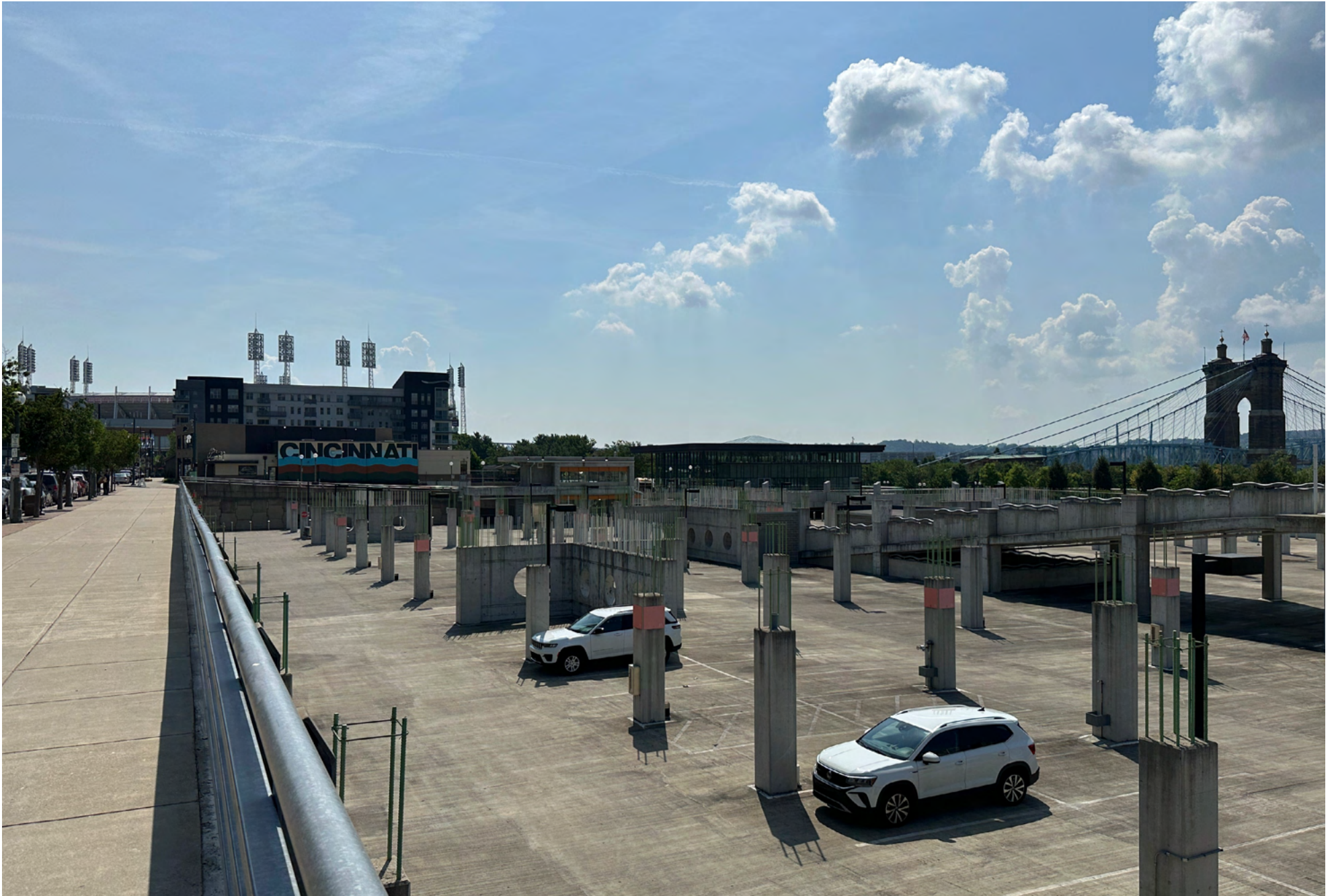
ABOVE Lot 24 looking toward Roebling Bridge
